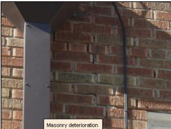
More mortar deterioration
