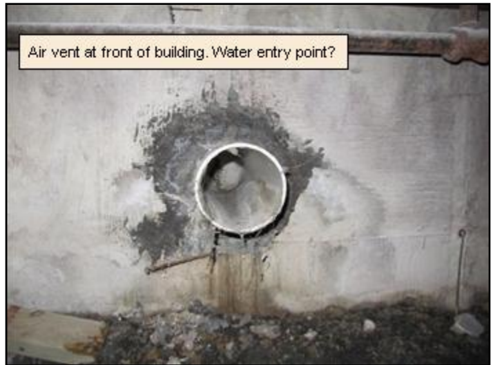
Water leakage in storage room
