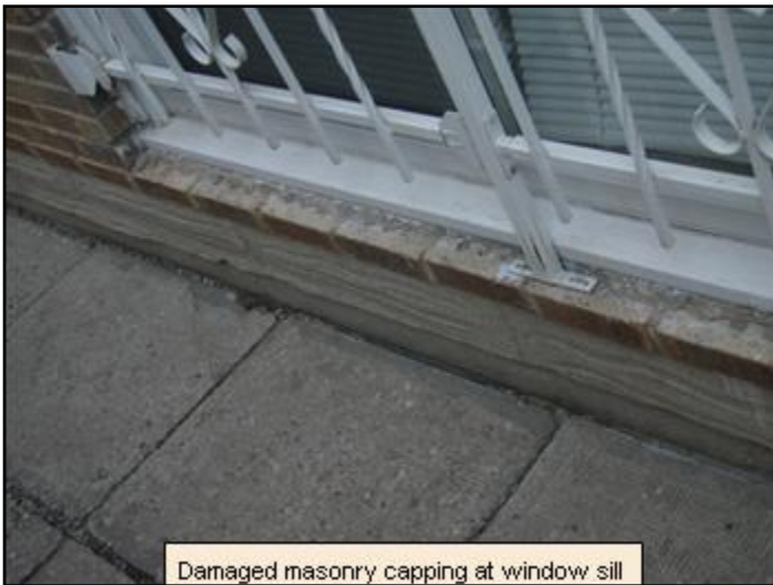
Damaged masonry capping at window sill
