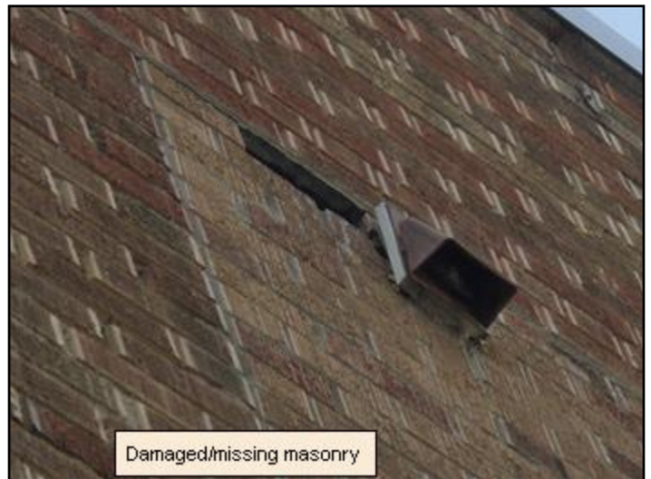
Masonry deterioration at window sill
