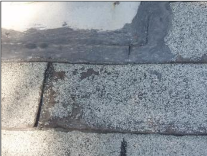
Garage roof at chimney
