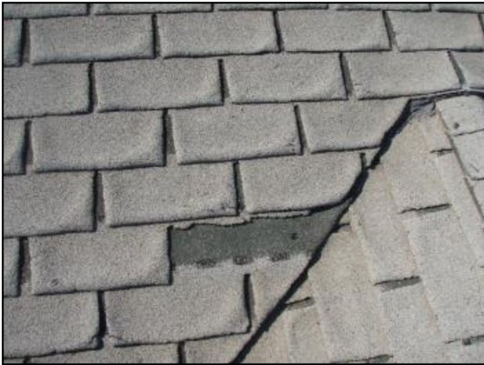
Damaged/missing shingles
