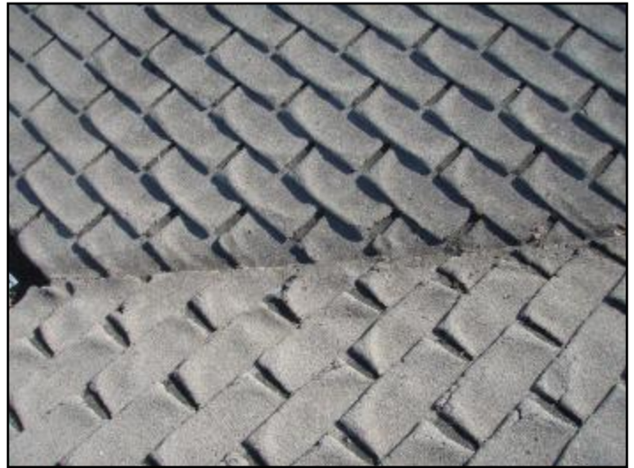
House roof north valley
