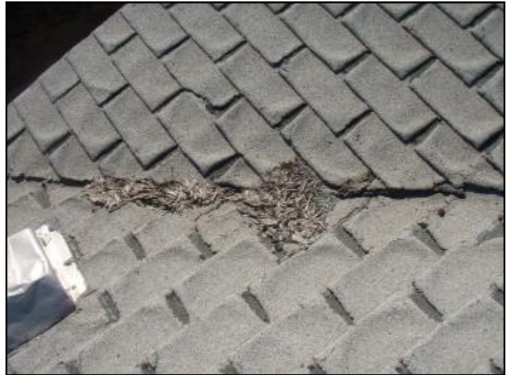
House roof south valley
